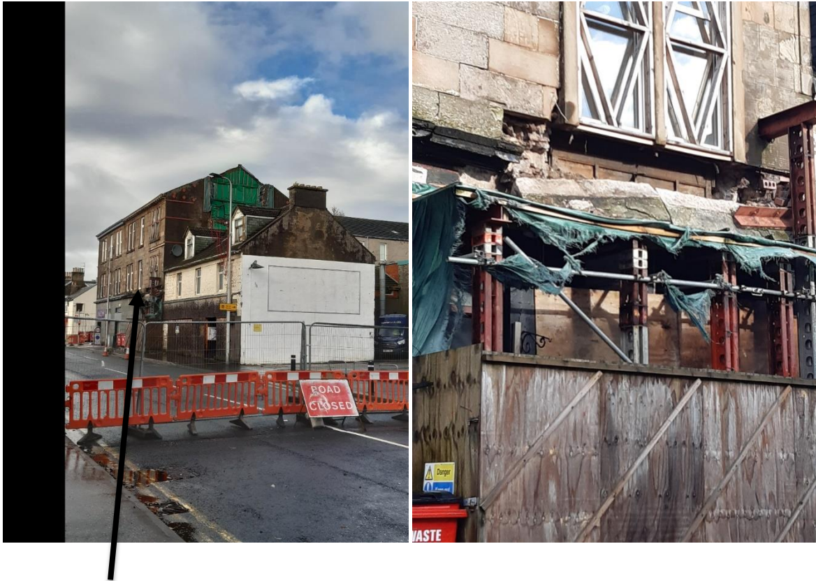
5-7 East Clyde Street- affected building
