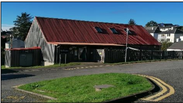
Tobermory Pre5 Unit has Energy Performance Certificate rated at Level 'A'
