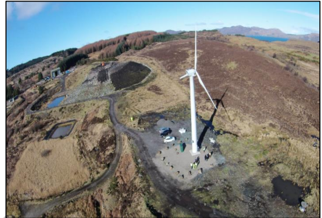
Council owned wind turbine @ Glengorm Landfill, Mull
