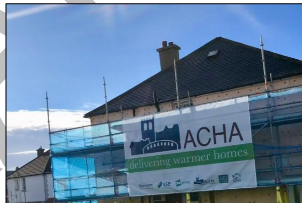
ACHA's External Wall Insulation works in Oban
